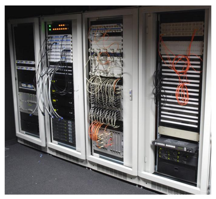
In the conference and banqueting halls mobile audio racks housing players and compact third-party mixers are available. These racks not only provide for flexible independent sound reinforcement, but also connect to the NEXUS network using a MADI board in the mixer. For security reasons, the operator can block the audio-network connection from the conference hall to prevent eavesdropping.
