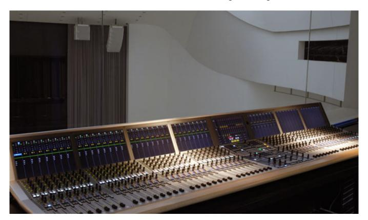
A STAGETEC CRESCENDO digital console with 56 faders, located in the large hall control room, and a NEXUS STAR router lie at the heart of the audio system. The console control surface can also be deployed in other locations in the house by connecting it to the STAR router via the optical cabling installed throughout the building. For example this enables the console to be used in the body of the hall . The audio-specific project requirements placed particular emphasis on equipment
