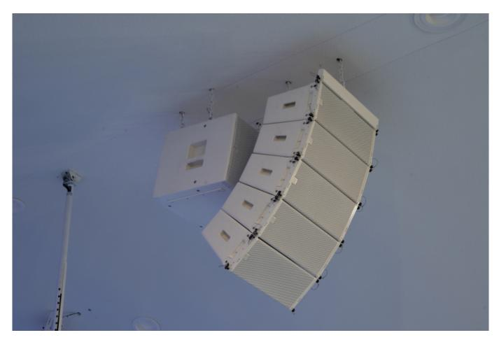
Zack Guida explained the thinking: "The roof is an A-frame, so we have set the array as high as possible. The flexibility to have one sub in the air, to ensure even coverage, and then a further two to provide high impact from the stage where necessary is fantastic. Further economies are achieved by being able to power the system from a single Martin Audio iKON iK42 4-channel process-controlled amplifier, configured in 2-box resolution.
