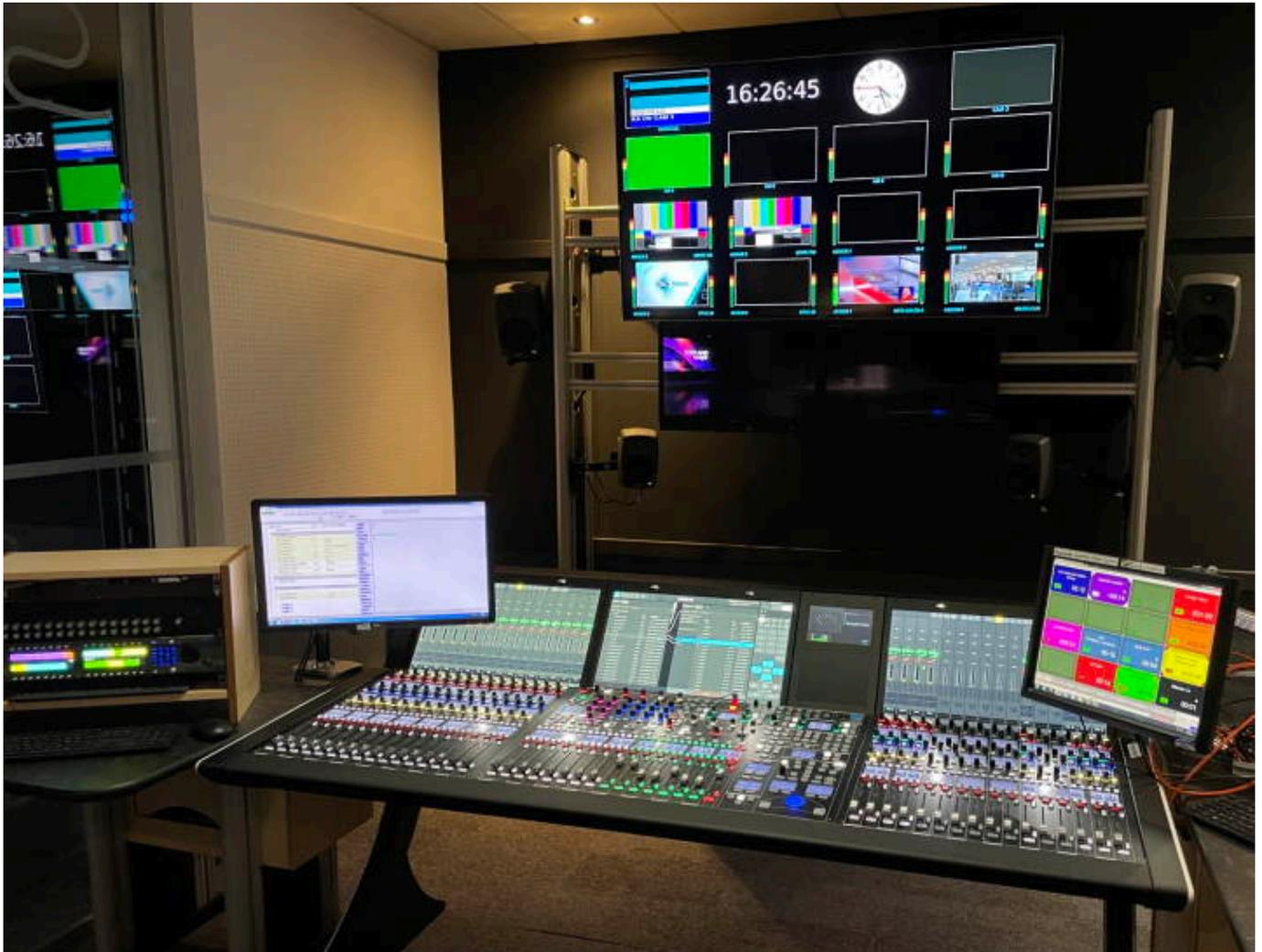
Scottish commercial broadcaster STV has undergone a full technical upgrade of its news production and sound control rooms and studio at its Glasgow HQ. Live programming is now on air, representing the UK's first on-air broadcast installation of Lawo's A\_UHD Core (Phase 2) and 48-fader mc<sup>2</sup>56 MKIII console. STV's broadcast channel reaches 3.2 million viewers each month alongside streaming service, STV Player, and STV Studios, Scotland's biggest production company.
